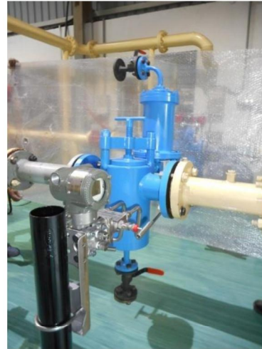
SAE with DP Transmitter
